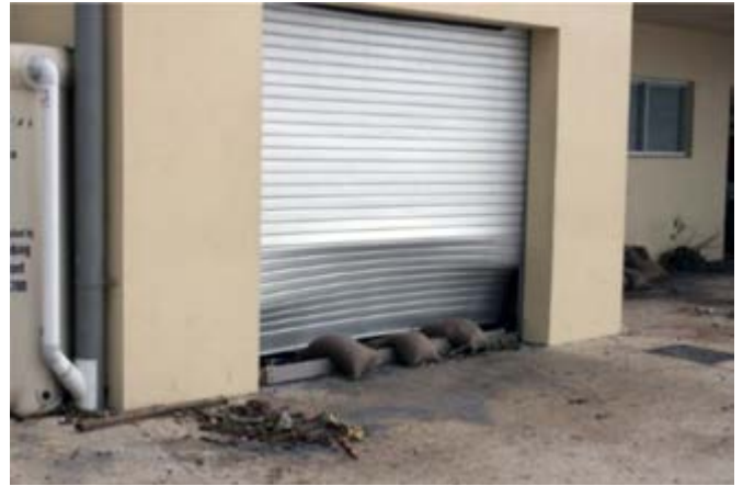
Figure 2 Examples of damage from coastal overwash at Terrigal Beach, NSW. This includes (left) damage to the Clan Motel adjacent to Terrigal Lagoon following the June 2016 east coast low, and (right) damage to the surf club roller doors at Terrigal after the same event.
