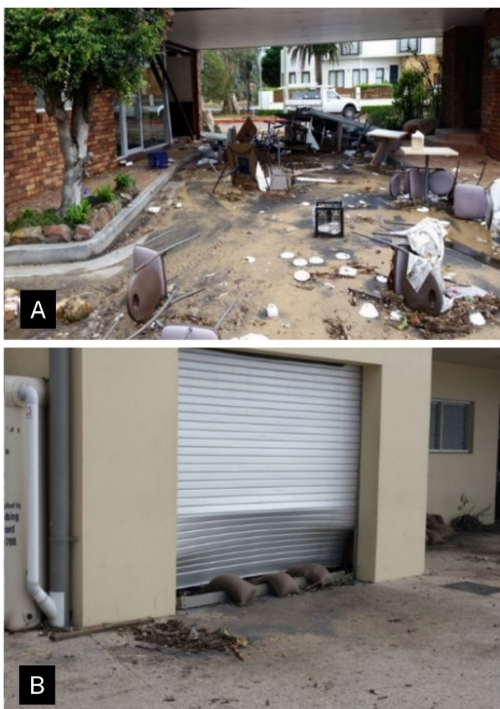
Figure 6 Damage resulting from overwash following the June 2016 East Coast Low at (a) the Clan Motel adjacent to Terrigal Lagoon and (b) the surf club roller doors at Terrigal Beach. Photos: DCCEEW
