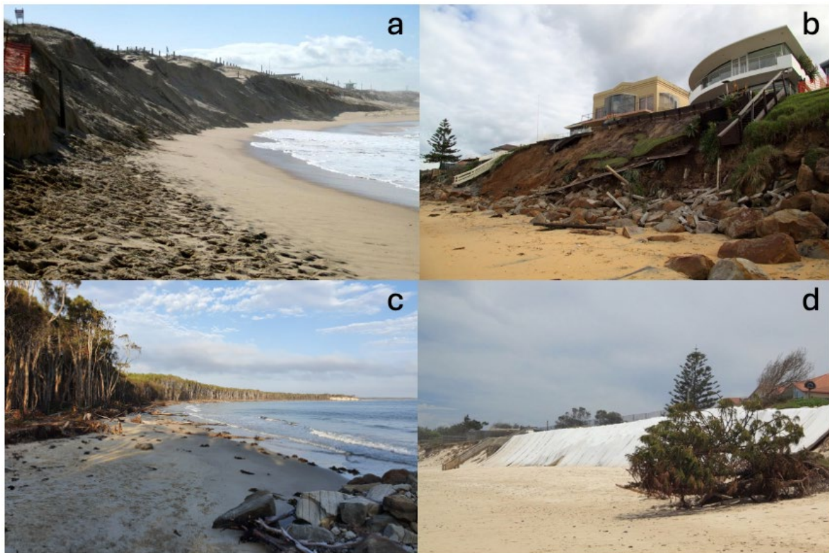
Figure 3 Fluctuating beach erosion caused by severe storm events in (a) an undeveloped setting at Cronulla and (b) a developed setting at Wamberal, compared with sustained shoreline recession in (c) a natural setting at Woody Bay and (d) a developed setting at Old Bar. Photos: M Kinsela
