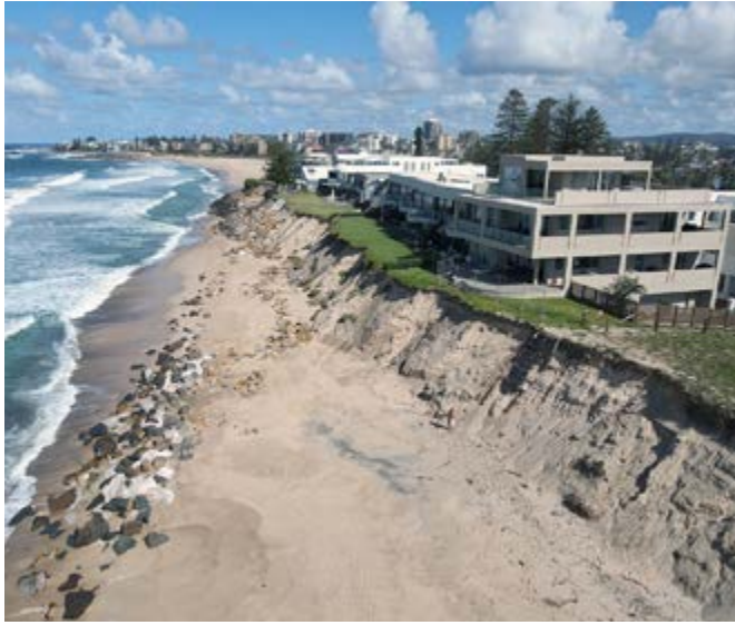
Figure 2: Coastal erosion of the dune at the Entrance North (left) and loss of structures at Wamberal (right).
