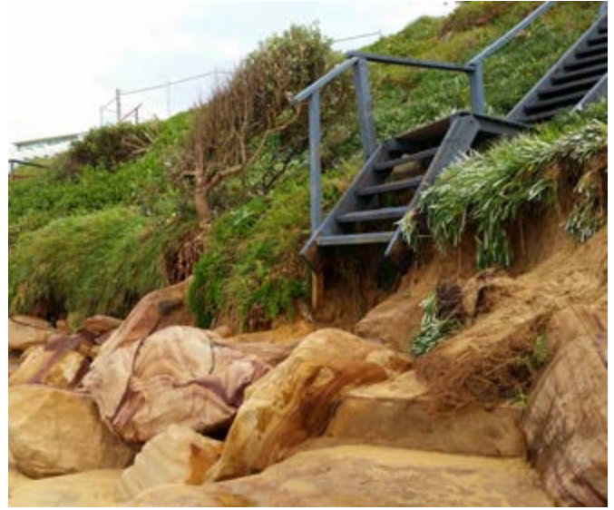
Figure 2: Coastal erosion of the dune at the Entrance North (left) and loss of structures at Wamberal (right).
