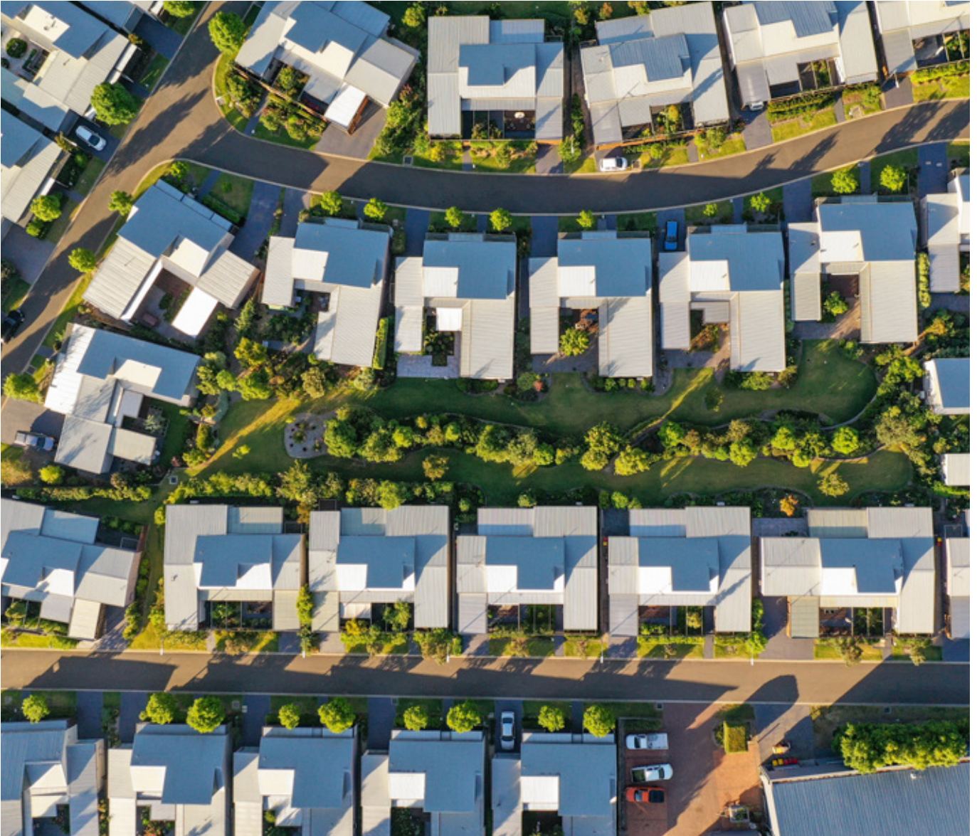
Aerial view of housing estate employing urban heat mitigation measures.
