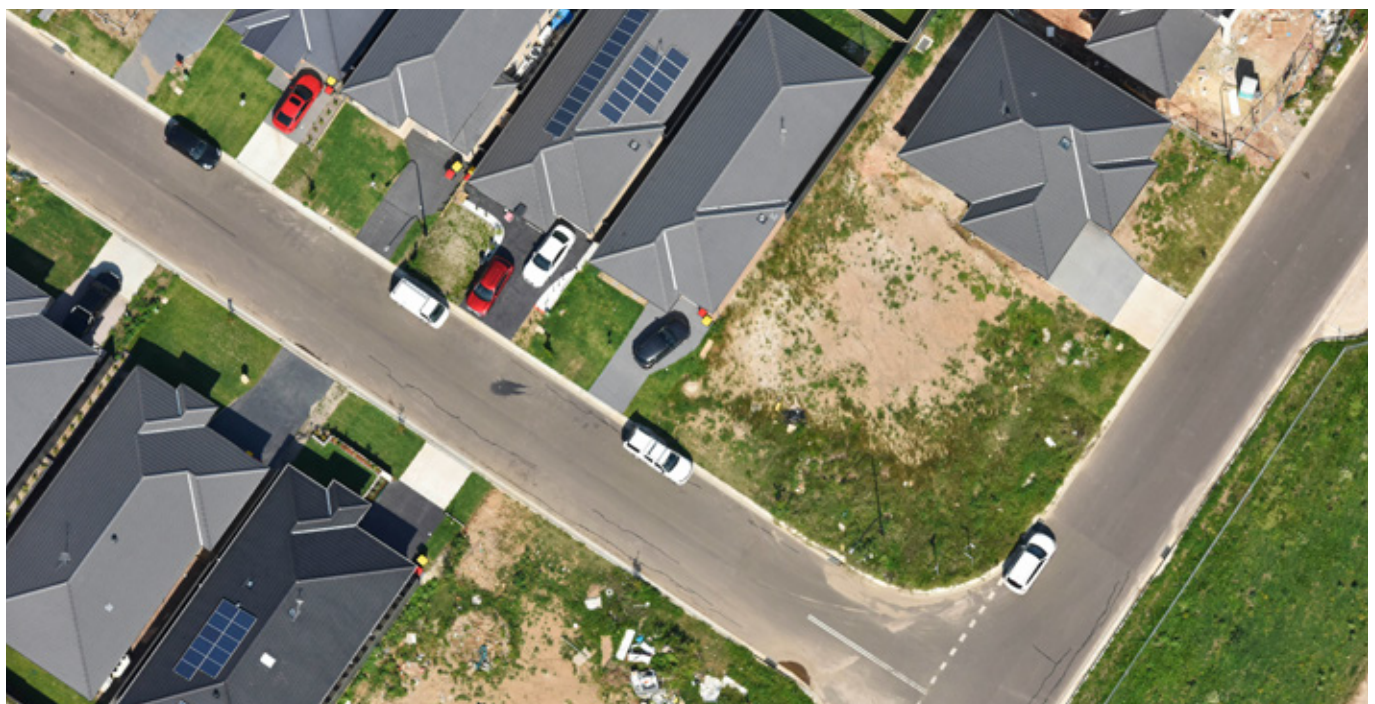
Aerial image of a new housing estate under construction.
