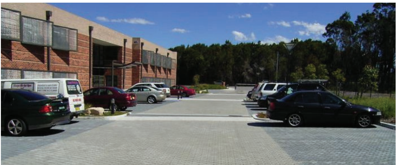
Permeable paving, Sutherland (Photograph: Courtesy WSUD.org)
