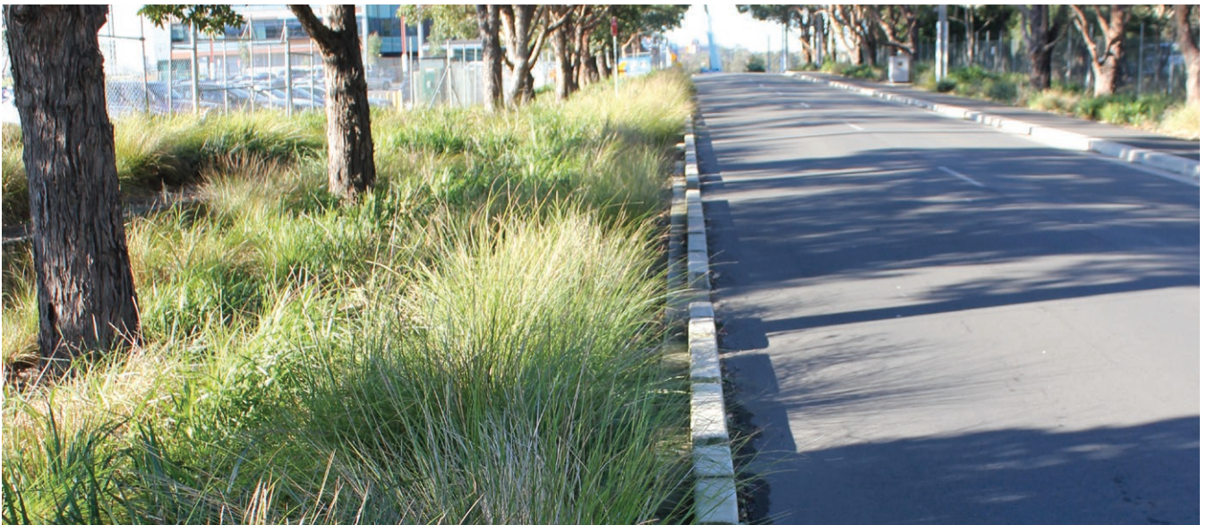
Bioswale, Sydney Olympic Park Authority (Photograph: Courtesy WSUD.org)
