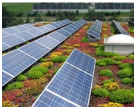
Solar panels have improved efficiency when used in combination with green roofs
