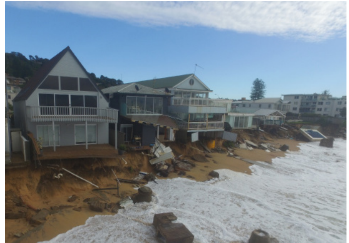
Collaroy-Narrabeen Beach storm erosion, June 2016 (WRL 2016)
